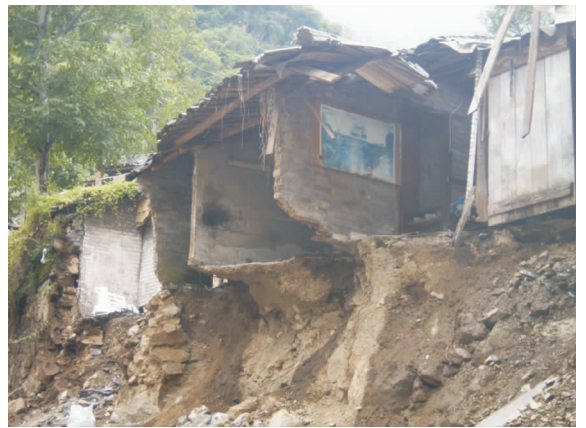
图6 2006-7-14 泥石流冲毁房屋 Fig.6 Houses destroyed by July 14, 2006 debris flow
