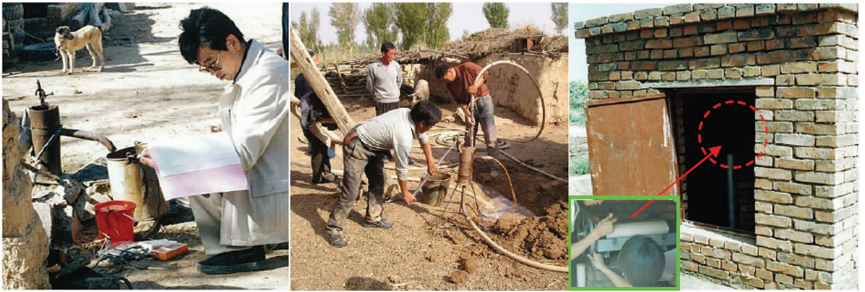
(Water quality survey Drilling operation Installation of observation well)
