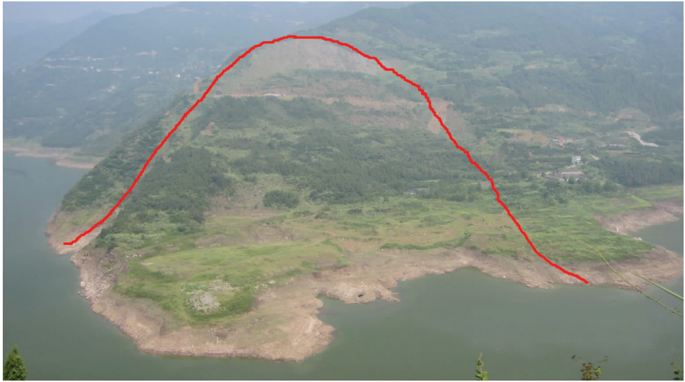
图 5 千将坪滑坡体全貌 Fig.5 Photograph of Qianjiangping landslide
