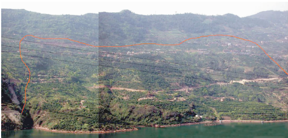
图 6 树坪滑坡体全貌 Fig.6 Photograph of Shunping landslide
