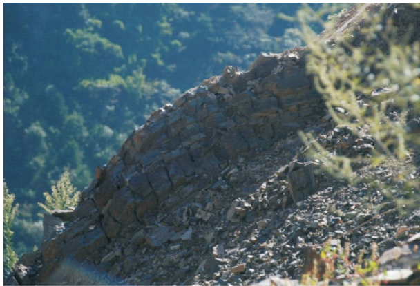
图7 剪出口右翼岩体弯曲隆起变形显著 Fig.7 Outstanding bending deformation of rockmass on the right of rockslide outlet
