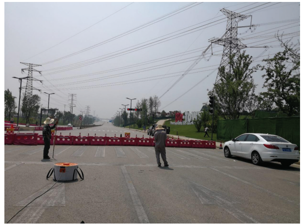
图7 研究区现场工况二 Fig.7 Working condition 2 of the test area
